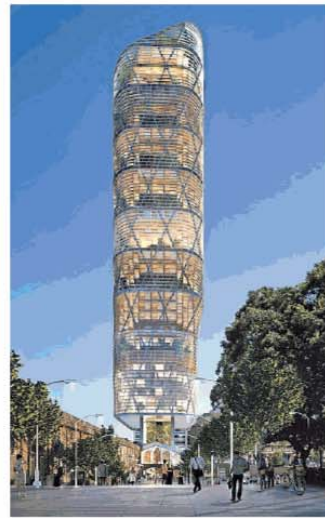
The 40-storey building has a concrete core but will use timber as the structural material on its floors.
